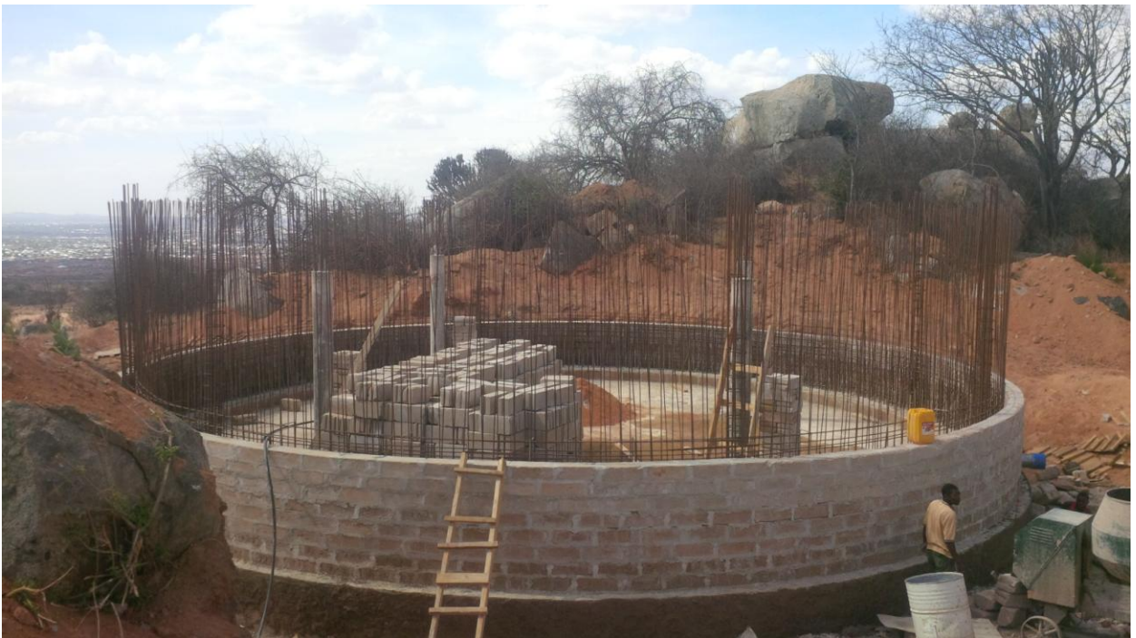
Formwork fixing for concrete wall
