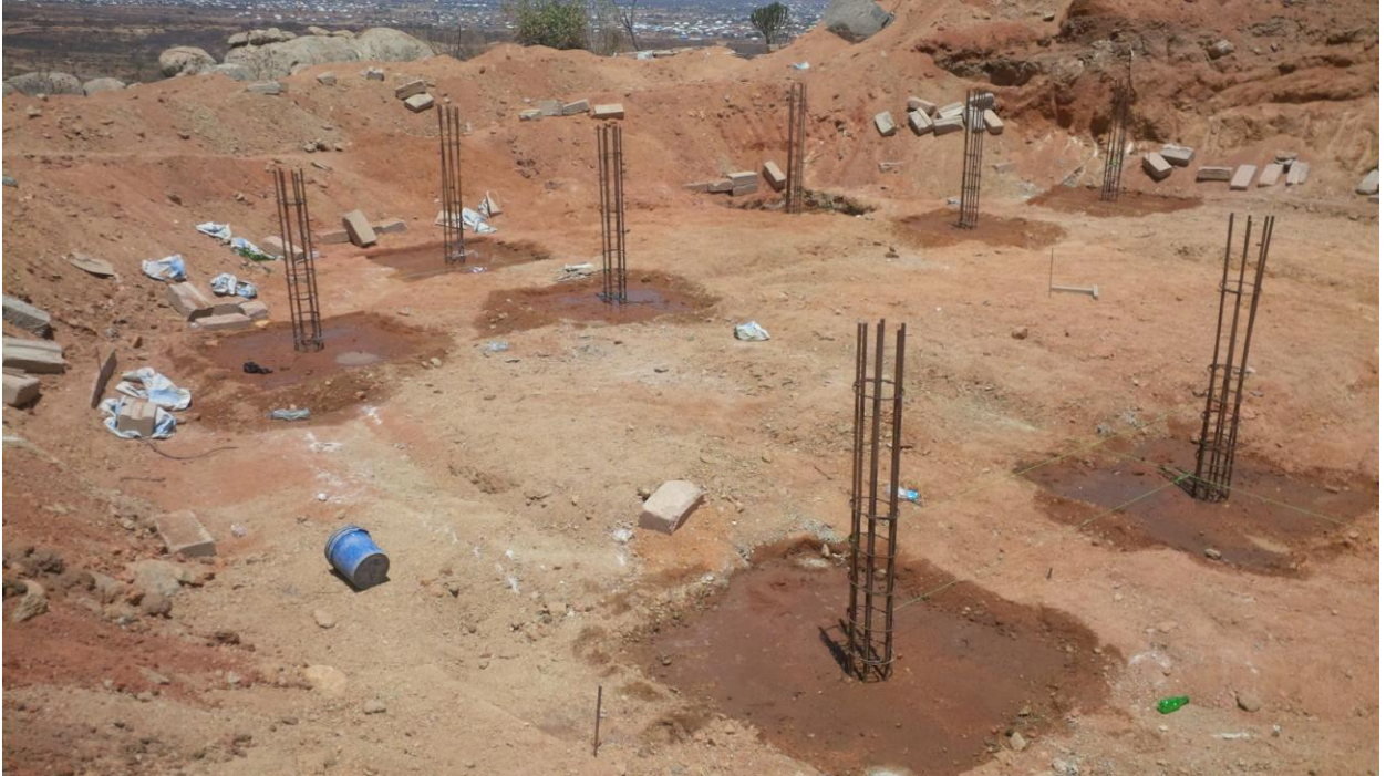
Preparation of foundation footings for water tank foundation
