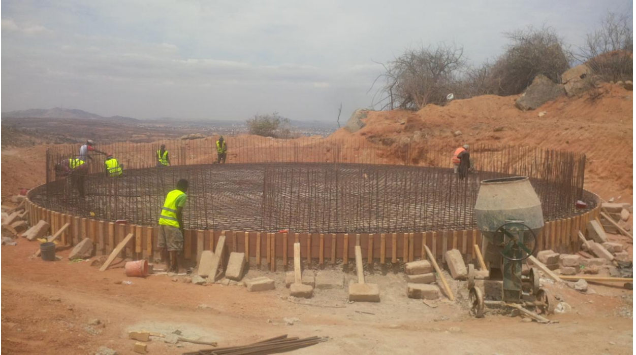
Steel fixing for the water tank base
